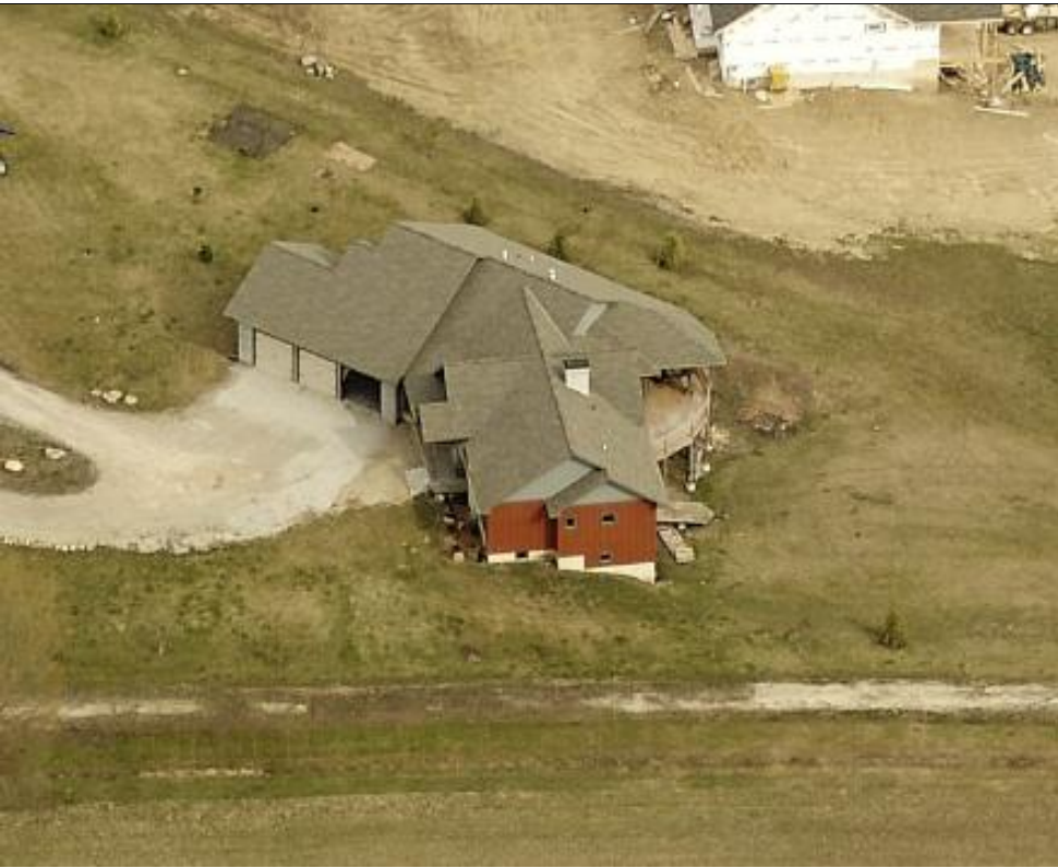
West Side View
