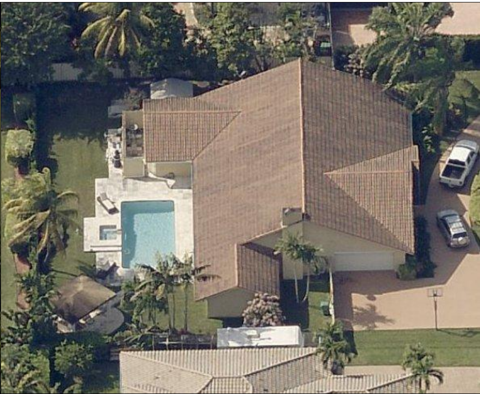
West Side View
